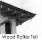
Wood Rafter Tail
