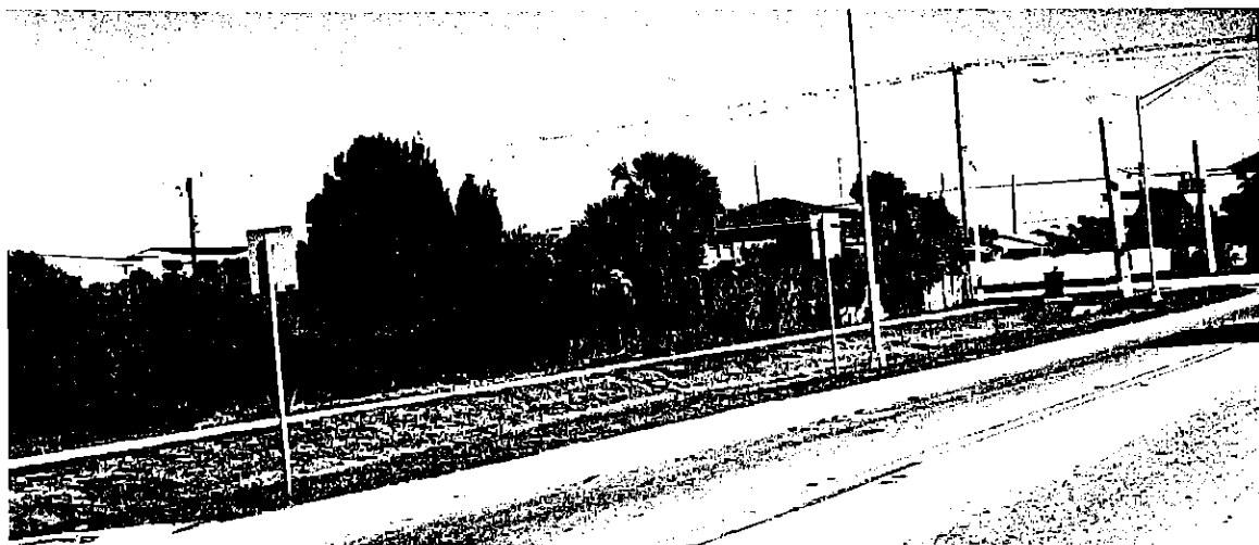
Location (B) NORTH SIDE OF EAST EXIT RAMP OF USINA BRIDGE
