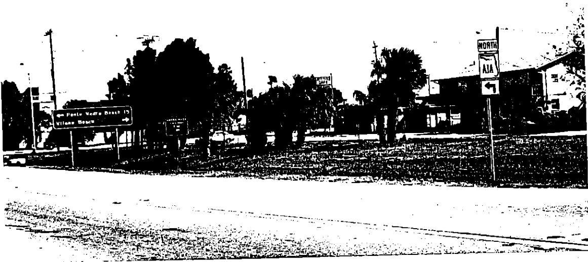
Location (C) SOUTH SIDE OF EAST EXIT RAMP OF USINA BRIDGE
