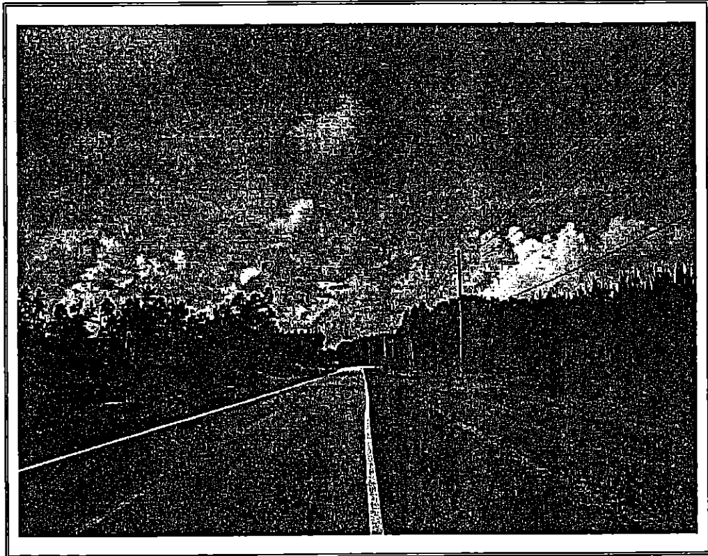
View of the Right of Way Looking South on CR 210
