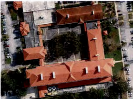
St. Johns County Courthouse East Annex-Roof Assessment
