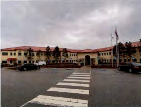
St. Johns County Health and Human Services 2nd Floor Renovation
