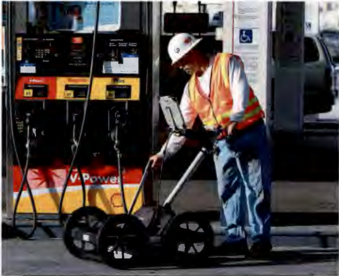
Marking fiberglass fuel lines with GPR
