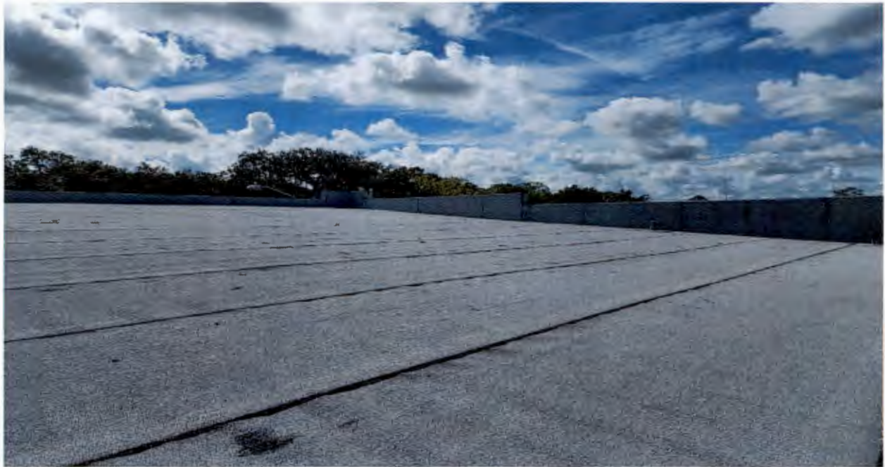
Photos 6 & 7: Flat roof
