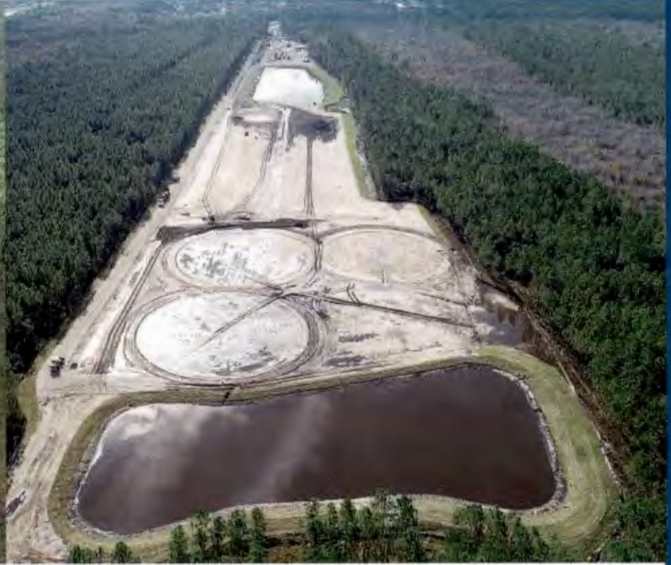
Site Conditions: December 5, 2023
