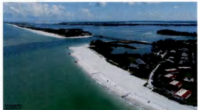
Year-1 post-construction condition of the structural stabilization and beach nourishment along the northern shoreline of Longboat Key. This project was identified as a high priority strategy in the 2019 BMP.
