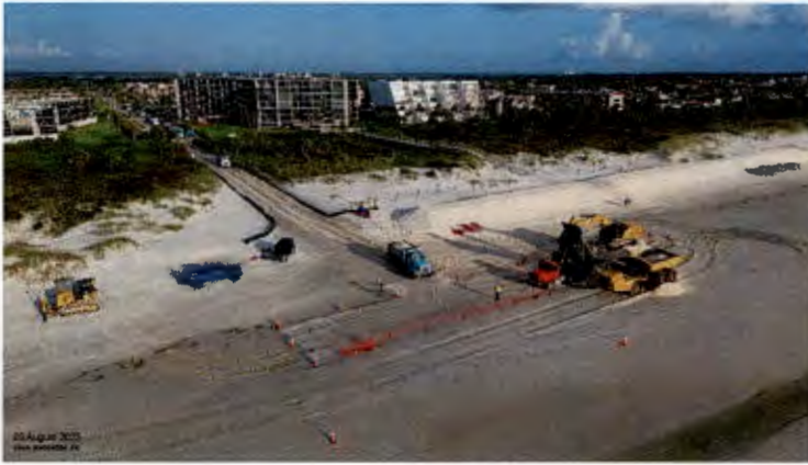
Figure 1 Truck haul emergency berm construction at Butler Beach on Anastasia Island (03 August 2023).
