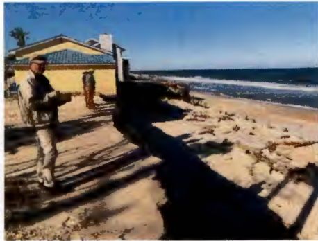
Beach Damage from Hurricane Ian, Crescent Beach (9/30/22)
