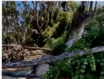
Pre-construction Eroded Conditions
