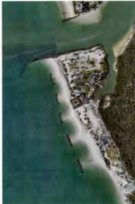
Keewaydin Island Erosion Control Structures
