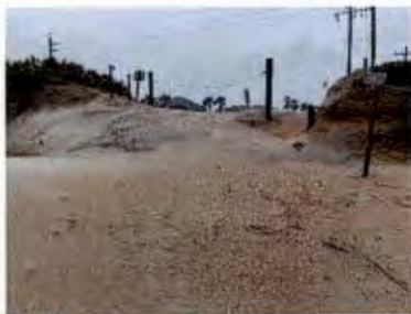
Pre-Construction Eroded Conditions
