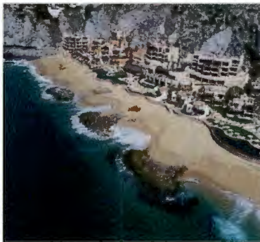
Constructed T-groins and Nourished Beach
