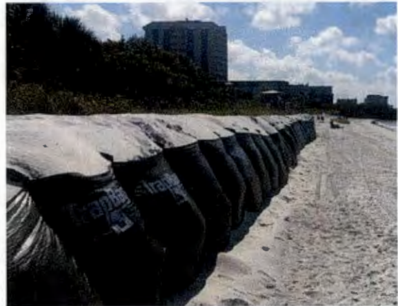
Trap Bag Installation in Volusia County, FL
