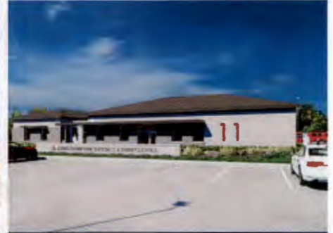
ST. JOHNS COUNTY FIRE STATION NO. 11 & SHERIFFS SOUTHWEST OPERATIONS CENTER
