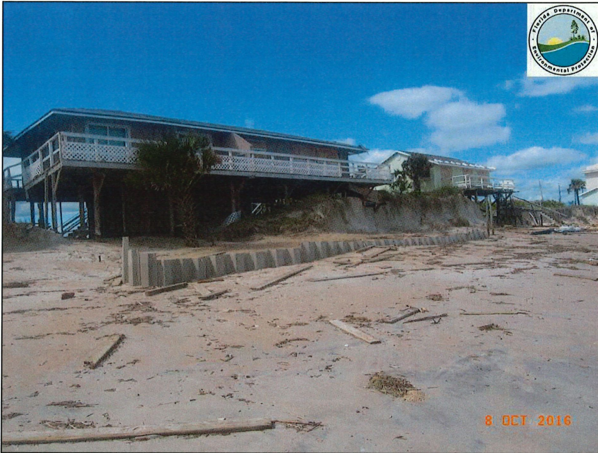
Figure 4-5. Hurricane Matthew damage in the vicinity of R116 on Oct. 8, 2016. Note top of vinyl sheet pile seawall emerging from sand in foreground and dune scarping and erosion below pile-supported homes. Image courtesy of Florida Department of Environmental Protection.
