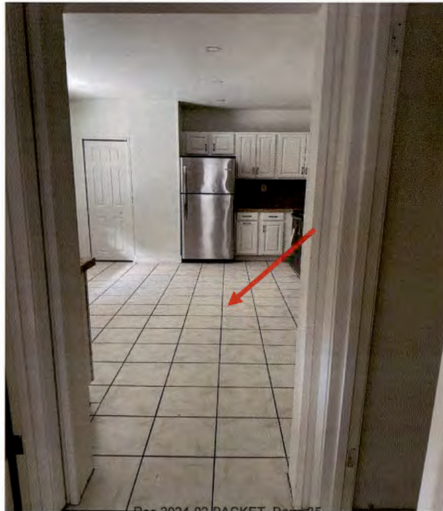
PHOTO 7-5: APARTMENT 1-KITCHEN, PRESERVED FLOORS: FACING WEST Updated version Received December 13, 2023 Planning & Building Department
