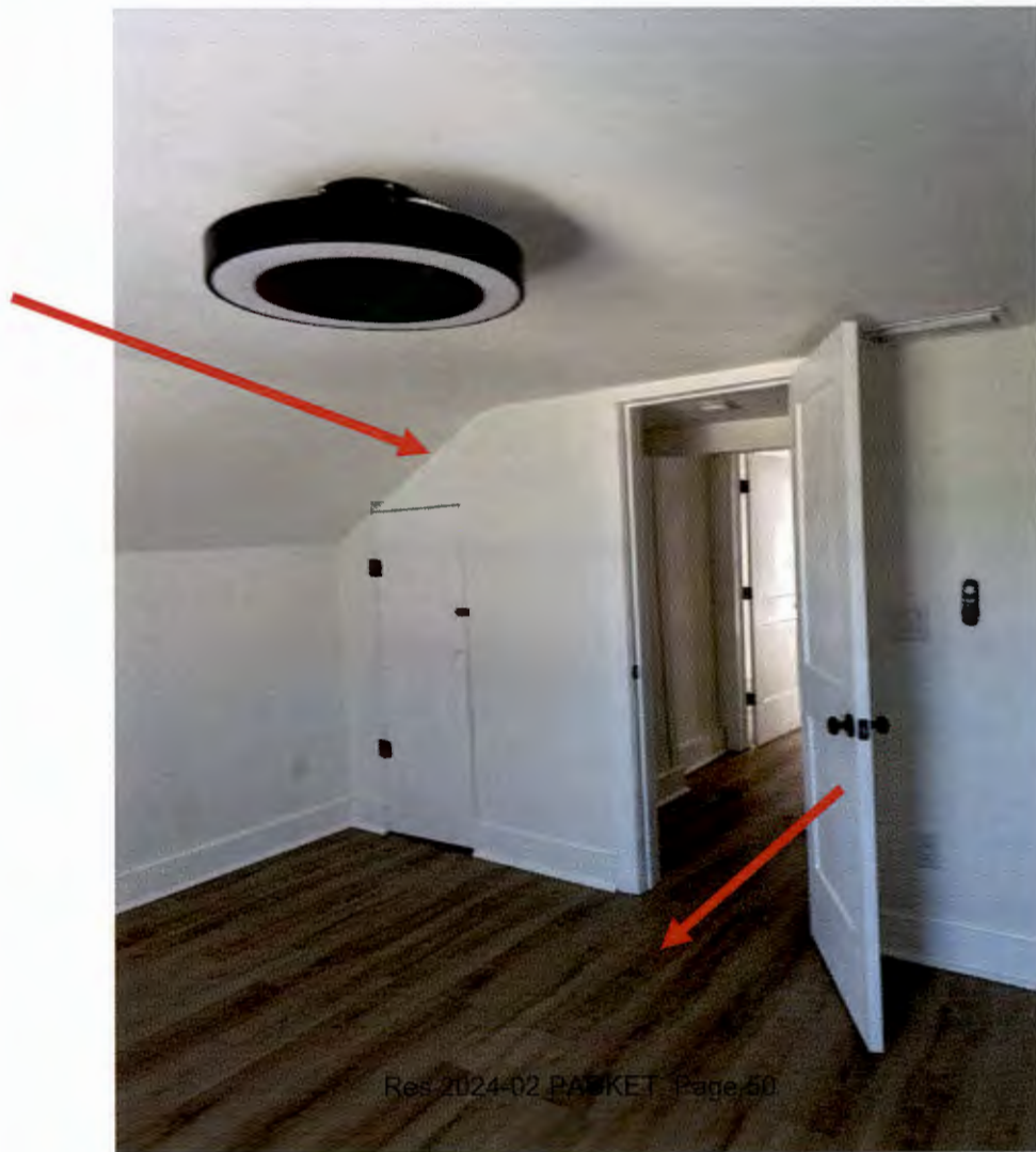
PHOTO 8-9: APARTMENT 2-BEDROOM, NEW FLOORS, HISTORIC WALLS. FACING SOUTH. Updated version Received December 13, 2023 Planning & Building Department
