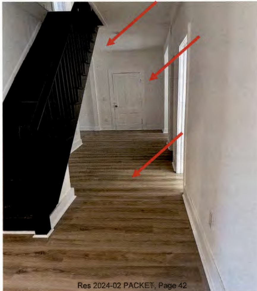
PHOTO 8-1: APARTMENT 2-HALLWAY, PRESERVED STAIRS, DOORS, NEW FLOORING : Planning & Building Department
