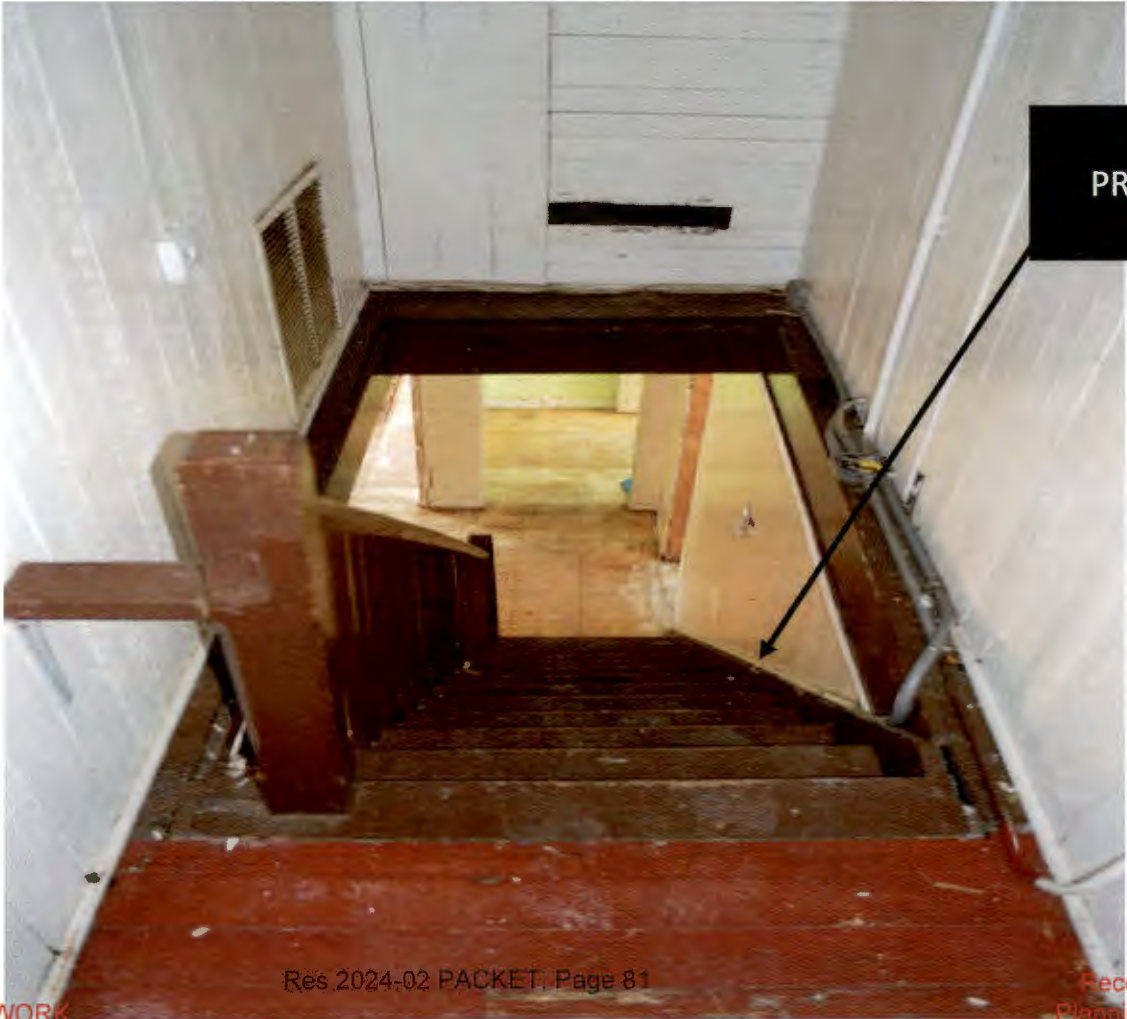
APARTMENT 3: 3rd floor, stairs, facing west
