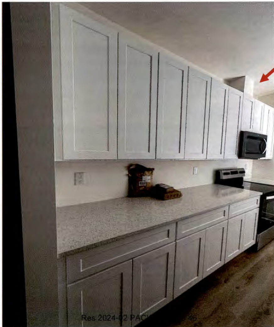
PHOTO 8-5: APARTMENT 2-KITCHEN, NEW CABINETS COVERING EAST WALL. FACING SOUTH. Updated version Received December 13, 2023 Planning & Building Department
