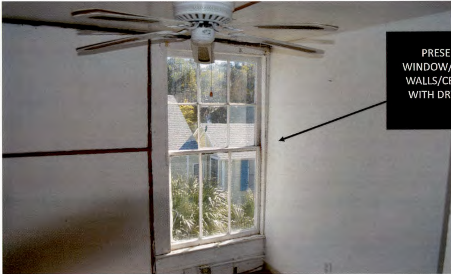
APARTMENT 3: 3rd floor, bedroom, window to be restored, facing south
