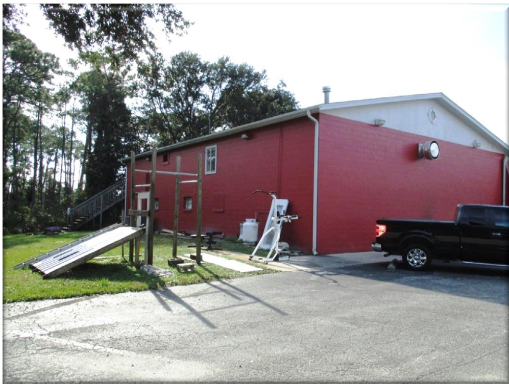
BACK OF BUILDING
