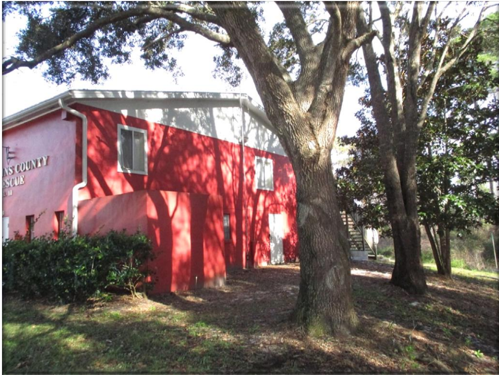
SIDE VIEW OF BUILDING
