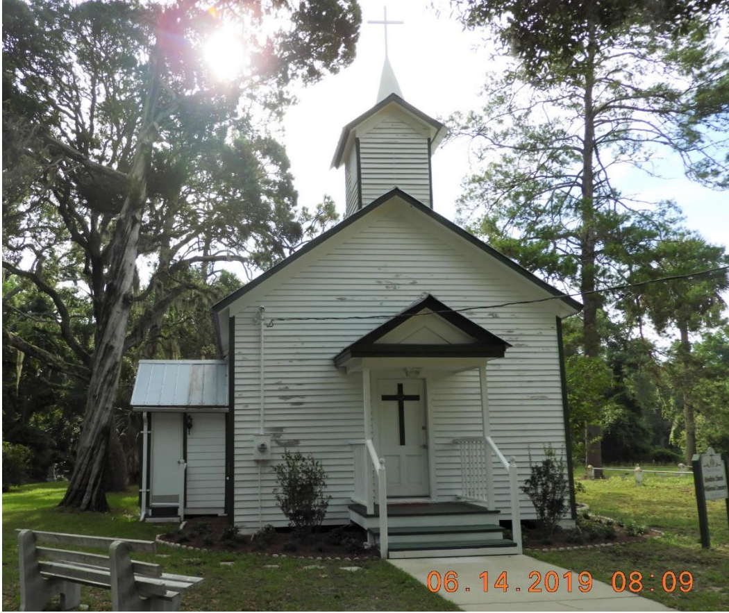
Figure 3 Moultrie Church front facade. Non-historic addition is adjacent, but not attached to north side of building.
