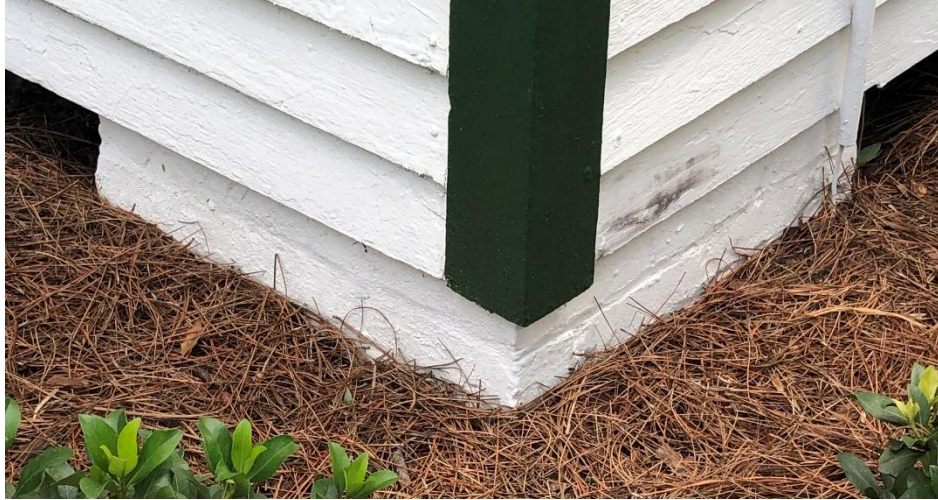
Figure 9 Close-up image of foundation.
