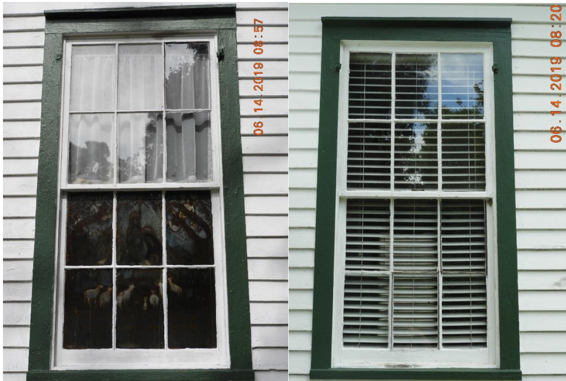
Figure 10 Left – Exterior view of painted window. Right – close-up of window.
