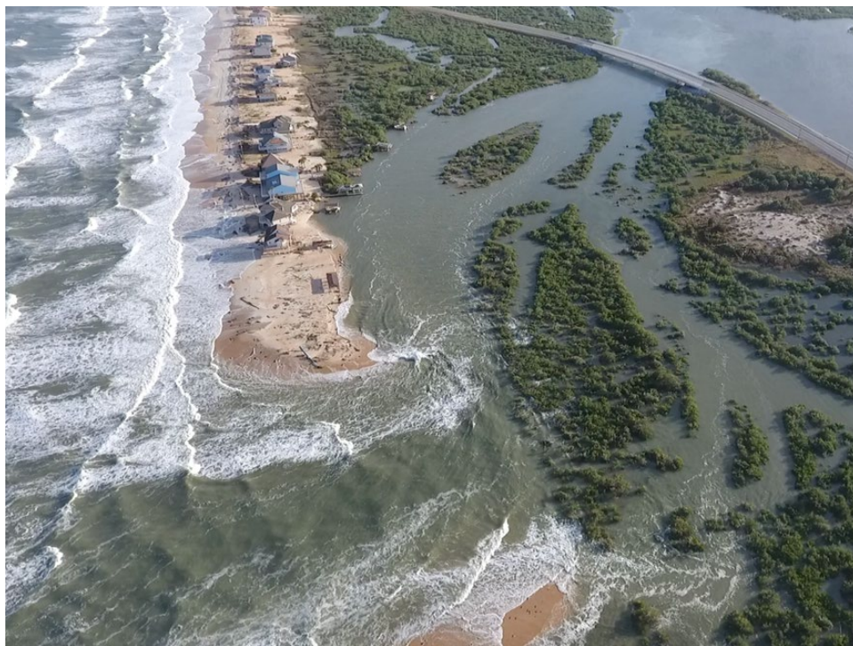
Figure 2.13 South End - October 2016 Breach Post-Hurricane Matthew (source: St. Johns County)
