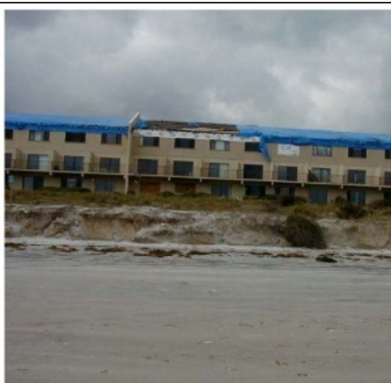
Photo 1 Anastasia Island Erosion at R-193
