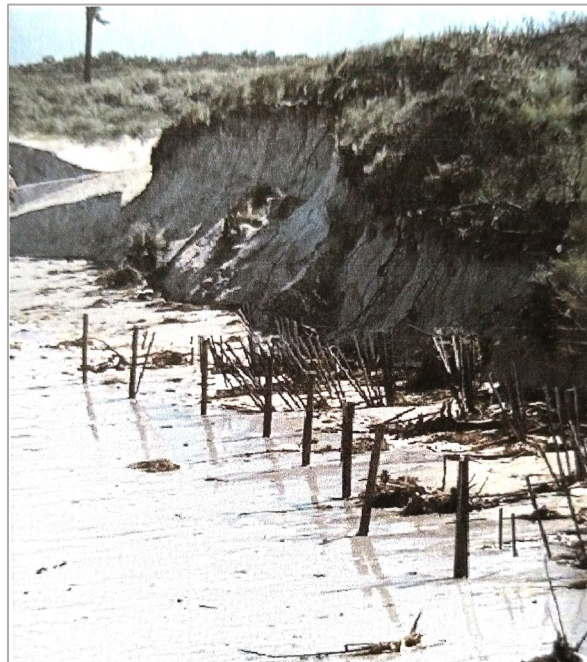
Figure 2.7 Post-Fall 2020 Northeaster Damage near Building 20 (source: Summerhouse)
