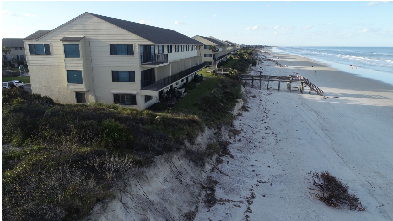
Figure 2.12 Post-Hurricane Nicole Conditions near Building 20 (Looking North) (source: Summerhouse)
