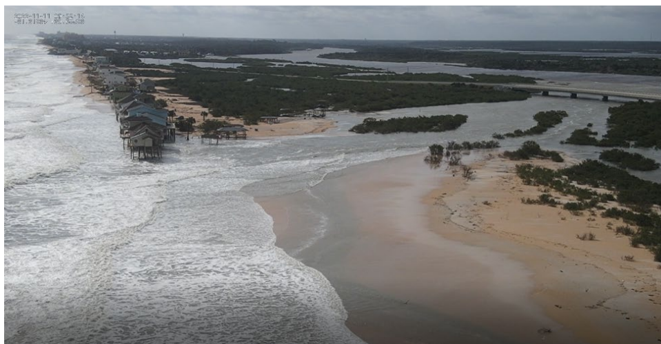
Figure 2.21 South End - November 2022 Post-Hurricane Nicole (source: St. Johns County)
