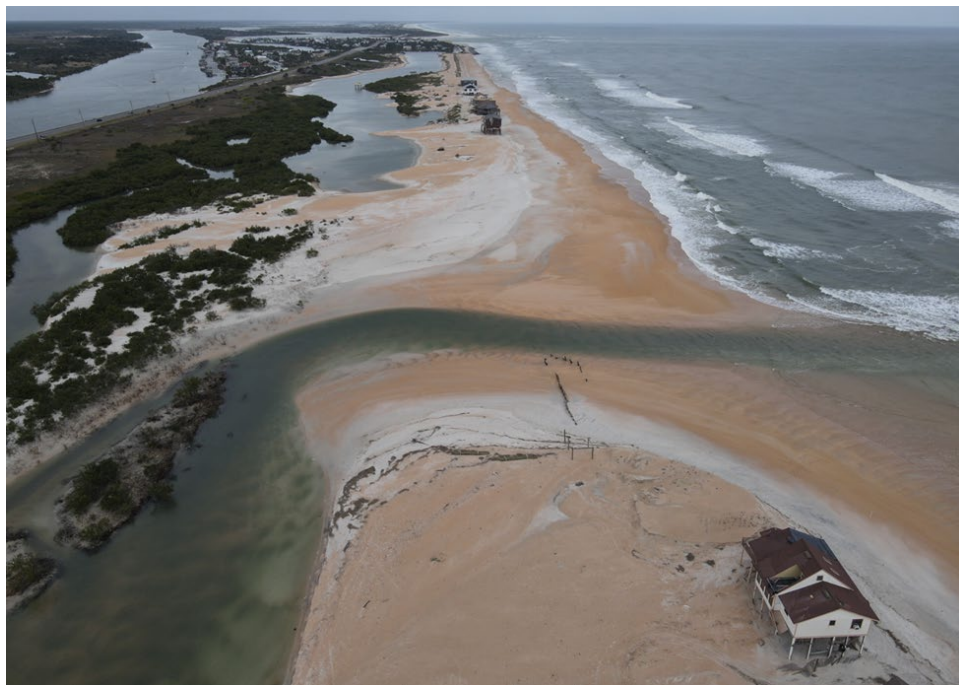
Figure 2.19 South End – November 2021 Post-Nor'easter (source: St. Johns County)
