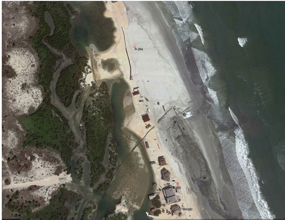
Figure 2.14 South End – March 2017 USACE/FIND Dredge Material Placement (source: Google Earth)
