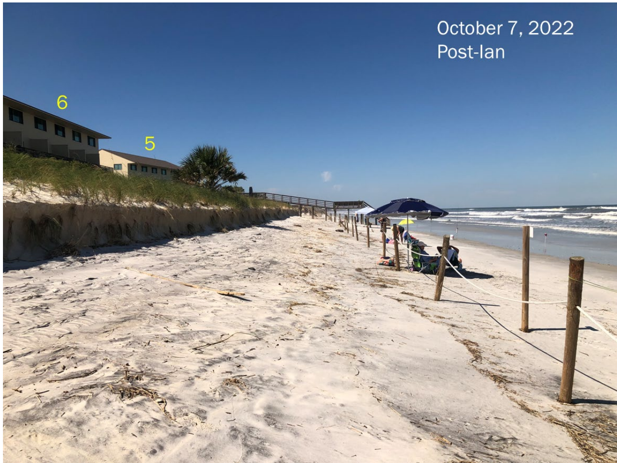
Figure 2.11 Post-Hurricane Ian Conditions near Buildings 5 and 6 (Looking North)
