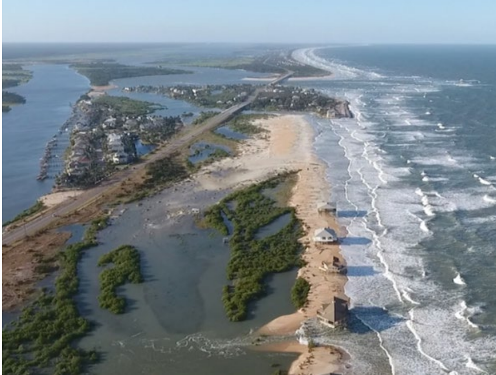
Figure 2.6 North End - October 2016 Post-Hurricane Matthew (Taylor Engineering, 2018)
