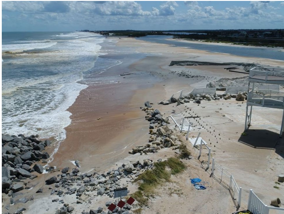
Figure 2.8 North End - September 2017 Post-Hurricane Irma (Taylor Engineering, 2018)
