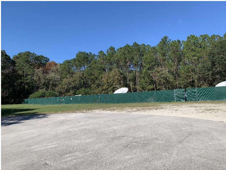
Camera facing northeasterly showing Pad 5.
