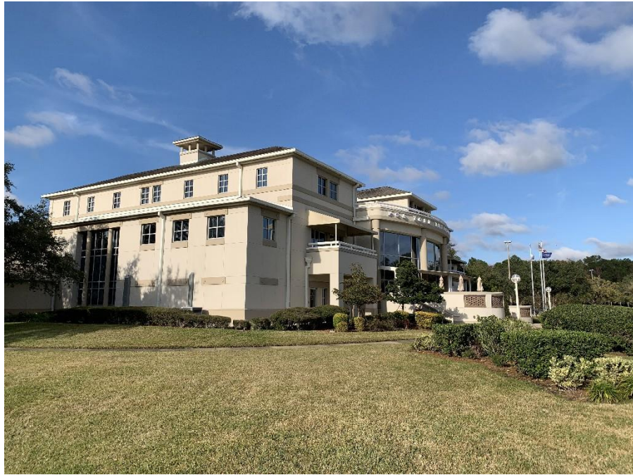
Camera facing northwesterly showing front of building.
