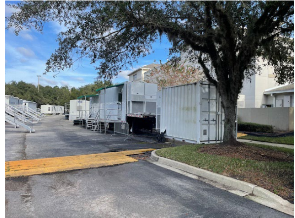
Rear View Office/Production Building
