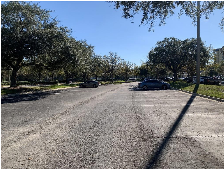
Camera facing southerly showing parking area.
