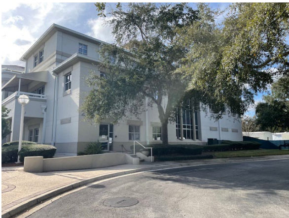
East View Office/Production Building
