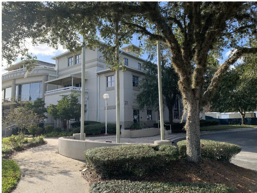
Camera facing southwesterly showing front of building.
